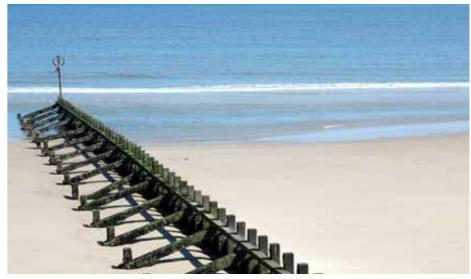
Image of the Groynes structures which are positioned along Aberdeen Beach
